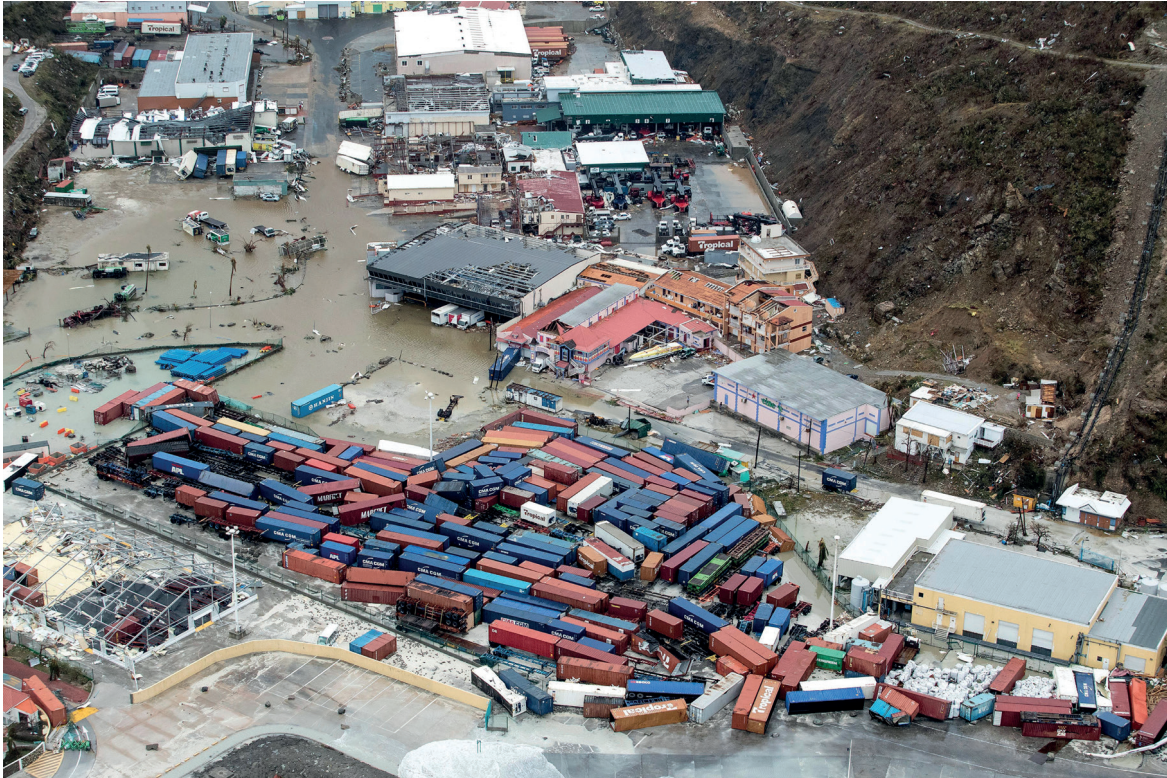
Photo: Overturned shipping containers in Sint Maarten
